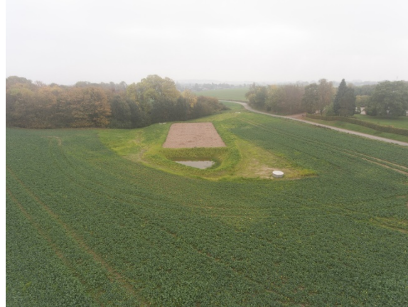
Constructed wetlands with woodchips
