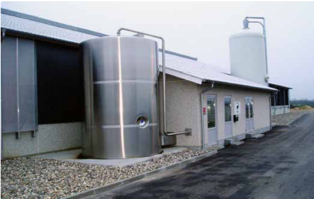
Fig 1. Outdoor located tank.
