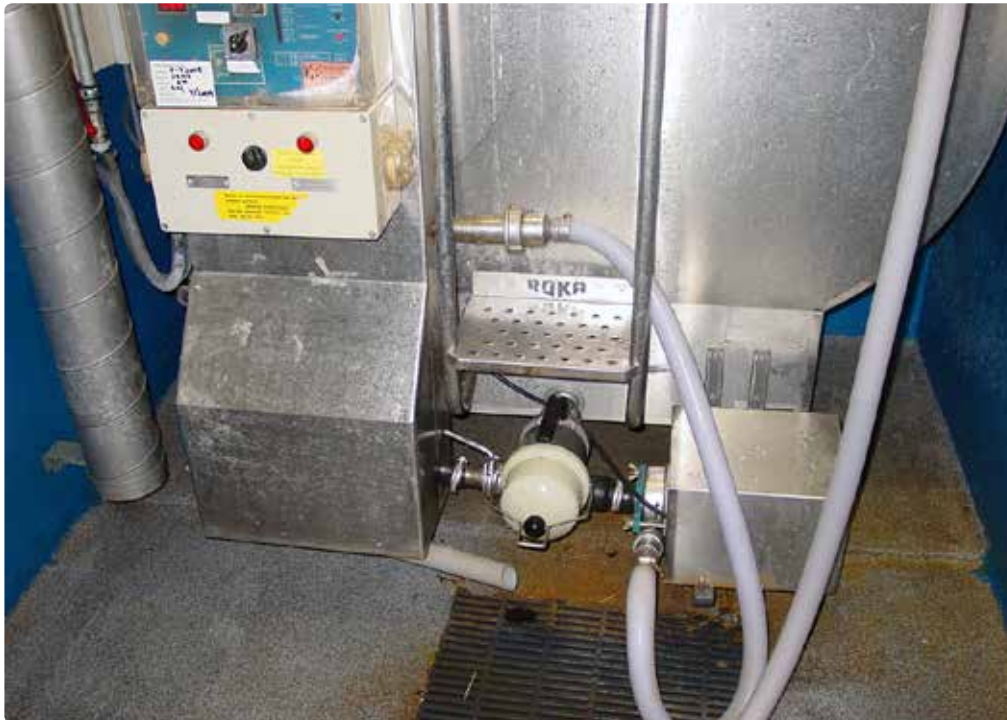
Fig. 2. Buffer tank conventional milking.
