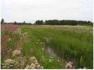
A two-stage ditch, with both flood plain on both sides.
