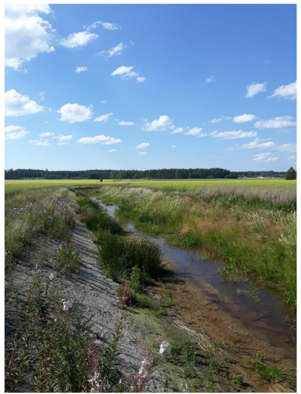
Pic. 2 A two-stage ditch, with one sided flood plain
