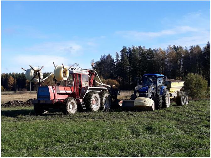
Pic. 3 Local sub surface drainage installation after renovation of the basic drainage
