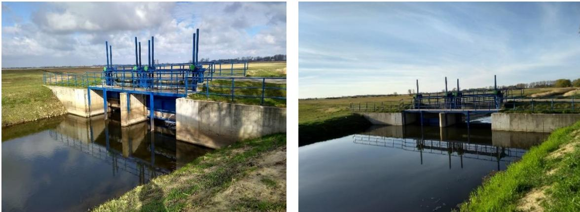
Photos. Damming water by hydrotechnical facilities, Moszczenica River, Bedlno Commune; the water is redirected to irrigation ditches
