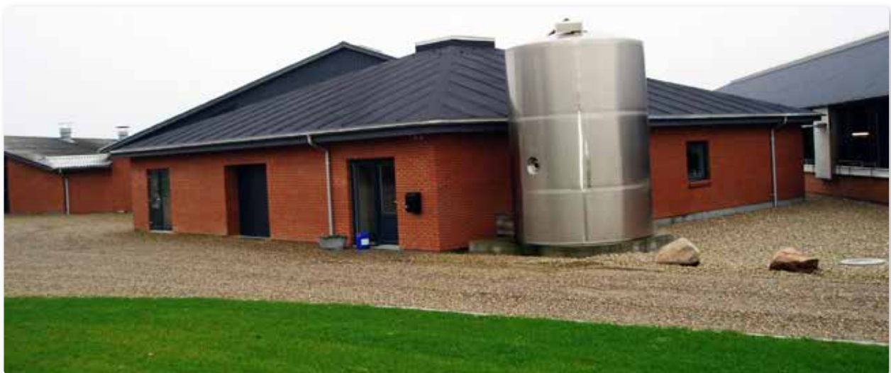
Detached service building containing milk room, equipment room and staff facilities.
