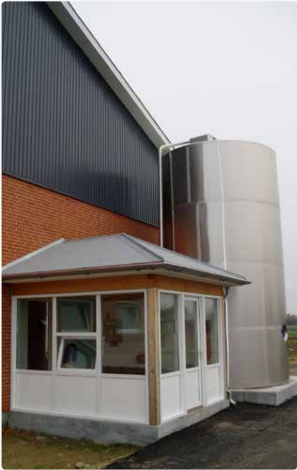
Silo tank placed at end wall of cowshed. Milk room in the form of dock, ensuring that the tank truck can drive directly up to the tank
