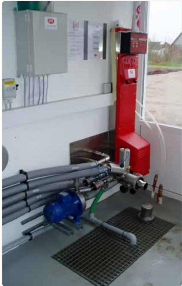
Acid-resistant floor drain with a stainless steel grate.
